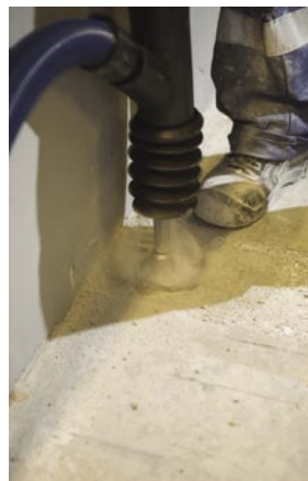
Drills and breakers can be coupled to dust extraction
