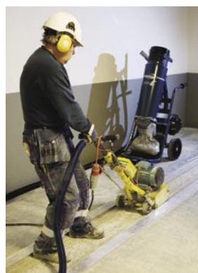
Surface preparation tools are often designed with inbuilt source extraction guards
