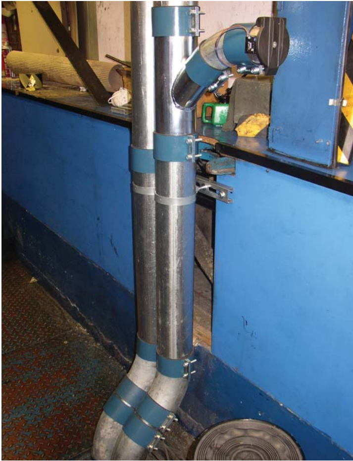
Cleanliness is a health issue: Extraction ducting is simplified by its modular components
