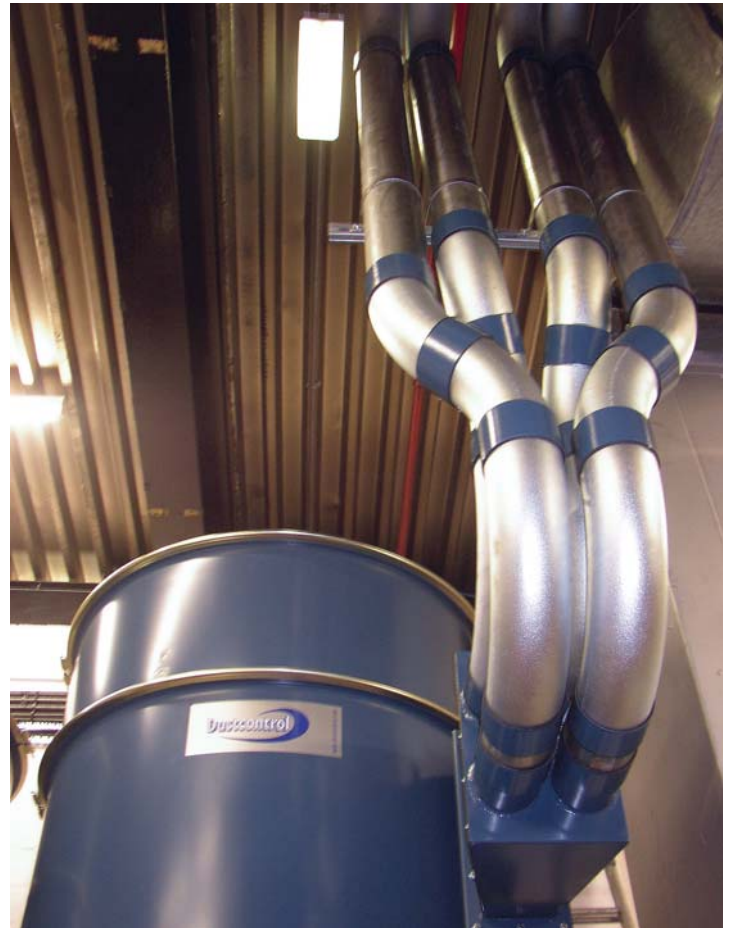
Cleanliness is a health issue: Extraction ducting is simplified by its modular components
